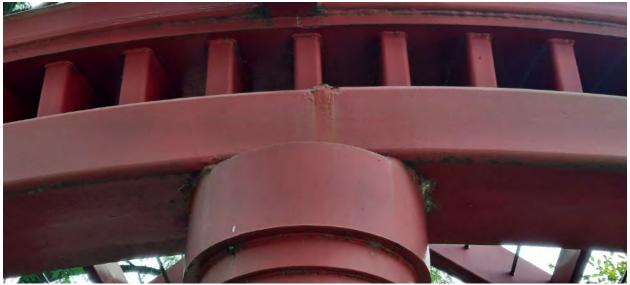
**6 Benches and 1 Can:** Remove from anchors, wash with degreaser, rinse, remove all loose paint, aggressively sand/grind rusted areas, sand remaining, surfaces, spot prime and coat all surfaces with automotive quality rust inhibitive spray primer (1 coat) and paint (2 coats), and remount. All per manufacturers specifications to achieve smooth, like-new condition. Color to match original.
