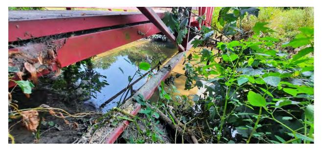
**Gazebo:** Wash with degreaser, rinse, remove all loose paint, aggressively sand/grind rusted areas, sand remaining surfaces, spot prime and coat all surfaces with automotive quality, rust-inhibitive spray primer (1 coat) and paint (2 coats). All per manufacturers specifications to achieve smooth, like-new condition. Color to match original.
