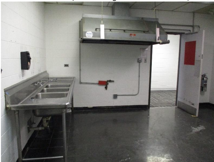
Kitchen (tile flooring has been removed)
