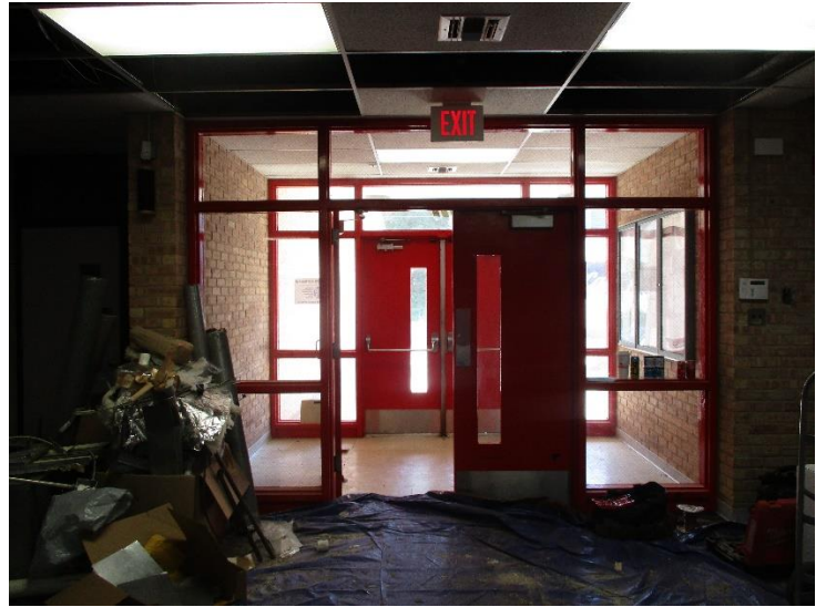
Front Foyer (tile flooring removed, flooring to be determined)
