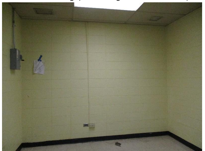
Kitchen Storage (tile flooring has been removed)
