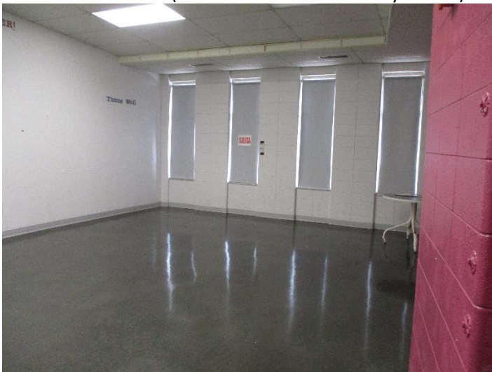
Classroom #7(tile floor to be removed by others)
