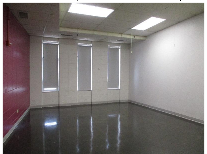
Classroom #8(wall in middle to be removed)
