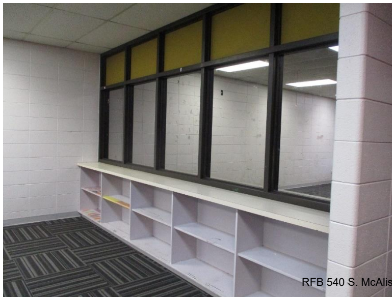
BOOKSHELVES IN CLASSROOMS TO REMAIN AND BE PAINTED. COUNTERTOP TO STAY AS IS. WINDOW TRIM TO BE PAINTED. YELLOW BOARDS TO BE PAINTED.
