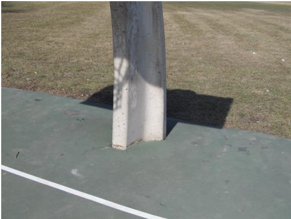
Minor delaminating
