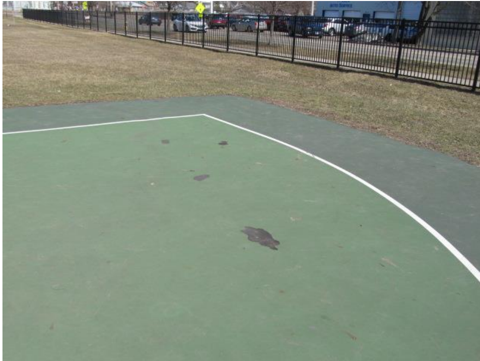
Minor delaminating
