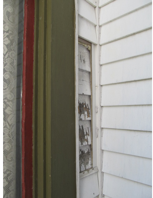
Fix siding with patching
