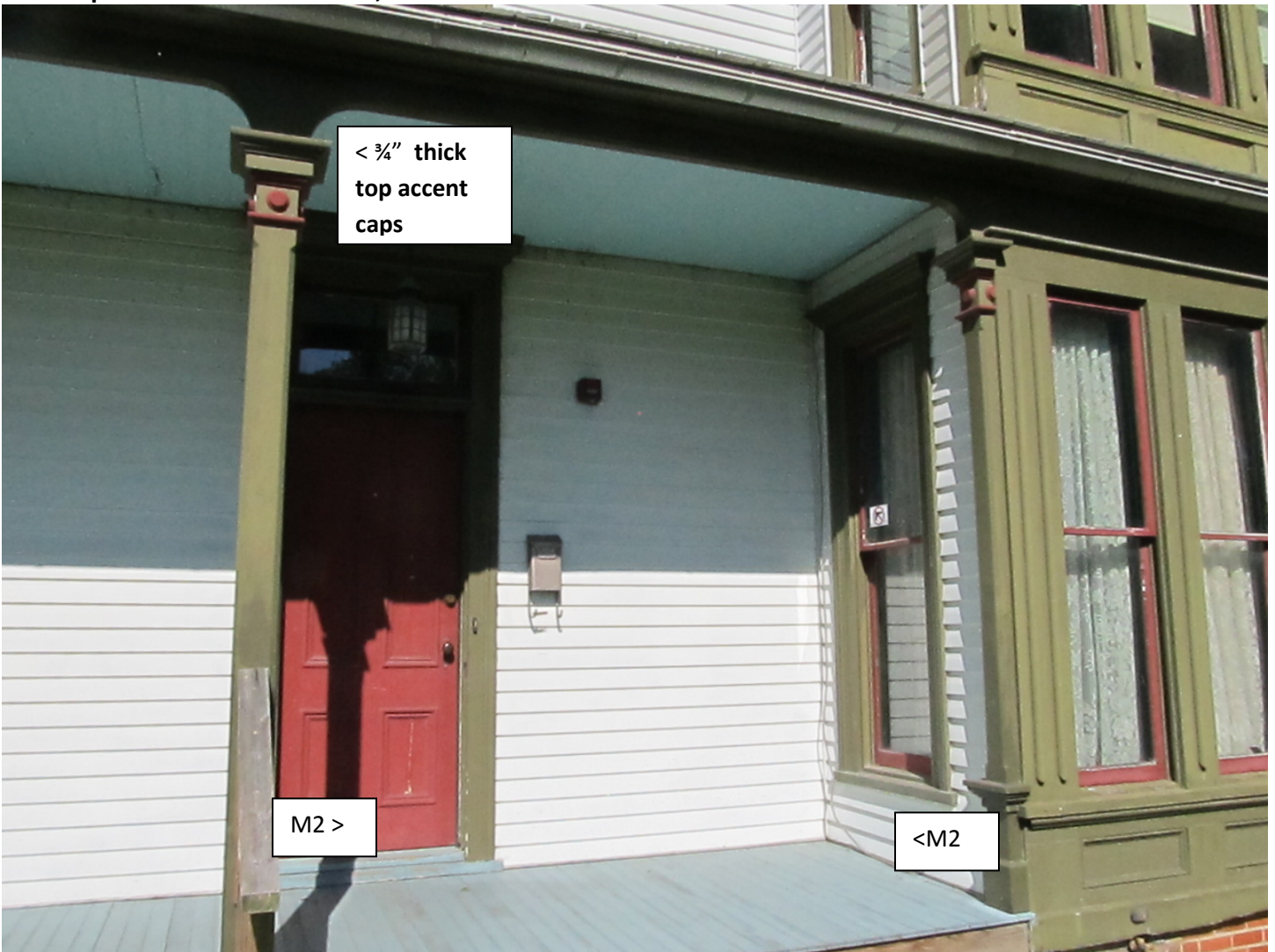
Mock-up 2 – to start at the door, include the area between the door and the window and the one window
