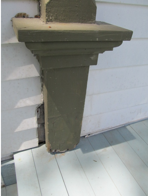
P10 – install aluminum siding and replace rotted 16” of wood post
