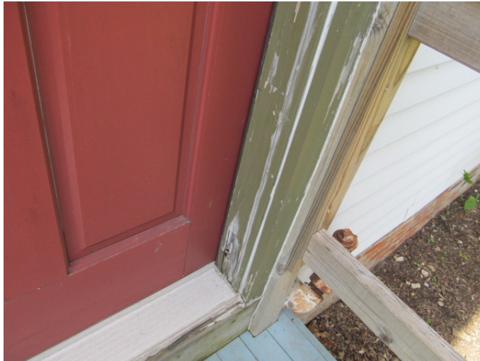
D5 – Replace rotted brick molding, replace bottom 16" of door jam.
