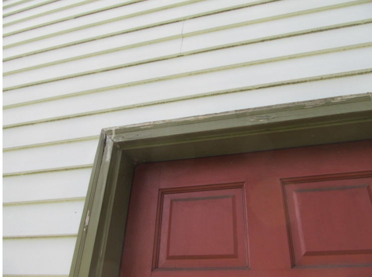
D5 – Replace rotted brick molding, install aluminum drip cap
