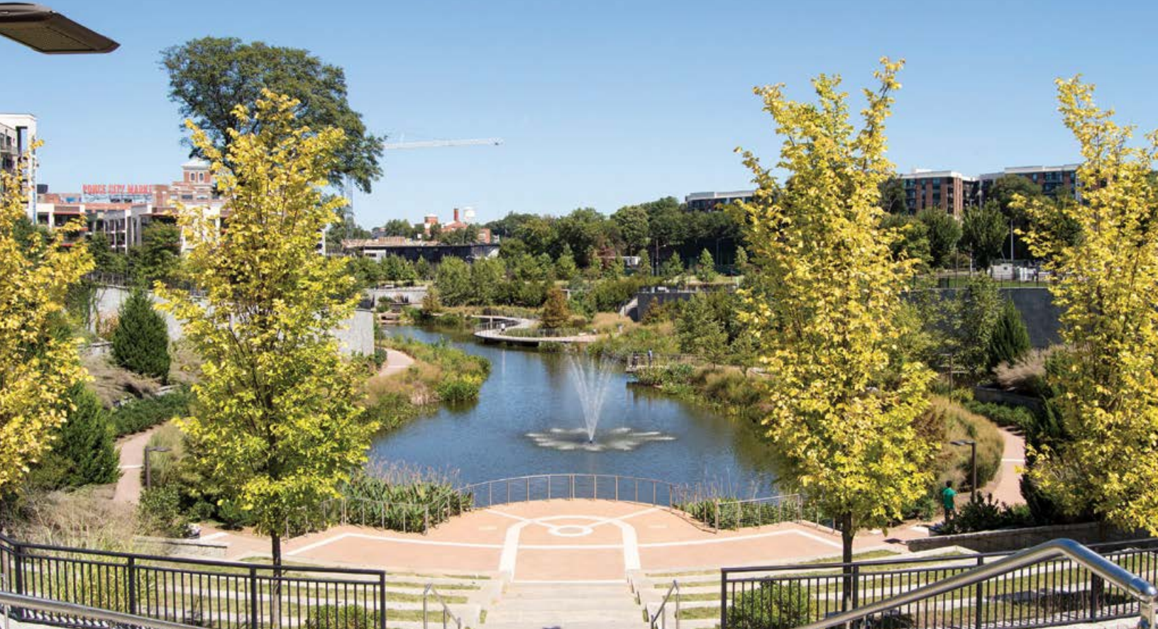
Historic 4th Ward Park in Atlanta, Georgia is a park that also serves as a stormwater retention system. Built in an area that has spurred much economic development, this park has become a model for others around the city and country.
