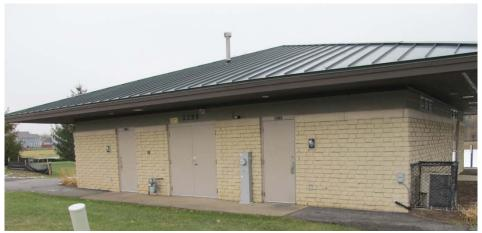
Spot prime doors and paint two restroom doors and utility door with gloss spray paint to match existing color. Brush paint or spray existing door jam and frames
