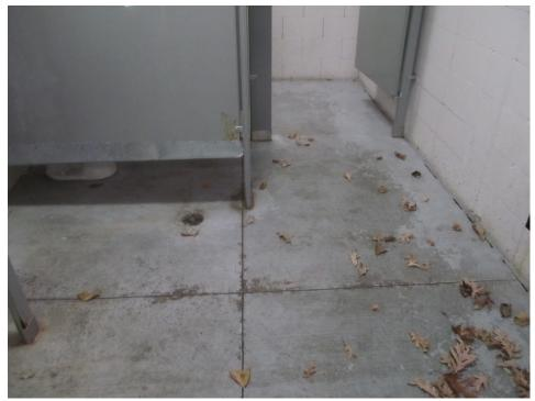
Fill cracks between the walls and floor with backer rod and install urethane based concrete caulk.
