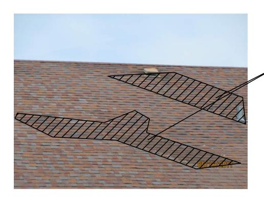
TWO AREAS OF MIS-MATCHED SHINGLES TO BE REPLACED TO MATCH EXISTING SEE ROOF PLAN FOR LOCATION
