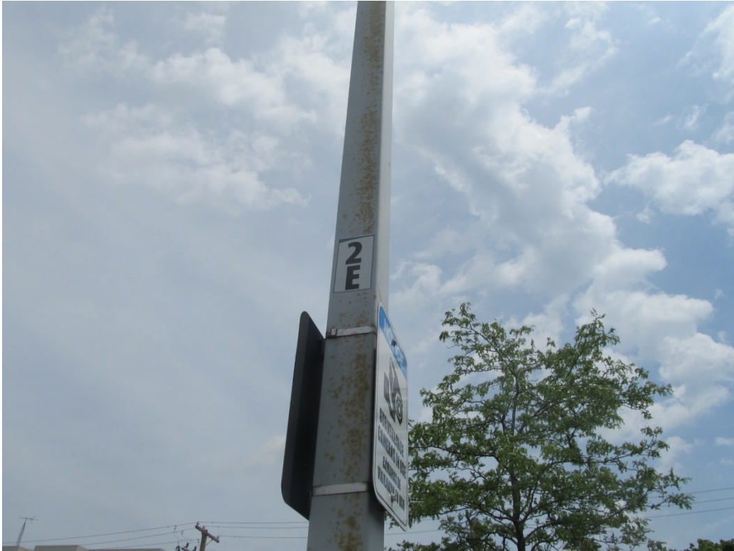
Signs to be removed and re-installed by contractor. Existing stickers to be painted around.
